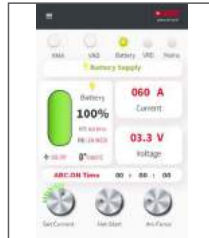
CONTROL & MONITOR BATTERY SUPPLY
