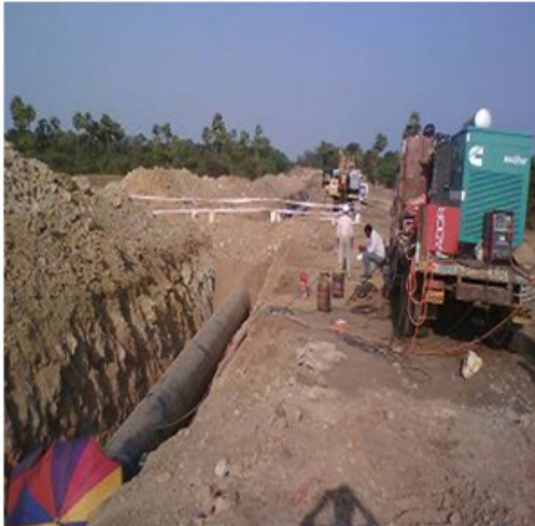
PAY LOAD OF 2 NO OF CHAMP MULTI 400 ON SITE
