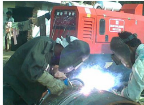
TWO WELDERS WELDING FROM OPPOSITE SIDES OF PIPE SIMULTANEOUSLY
