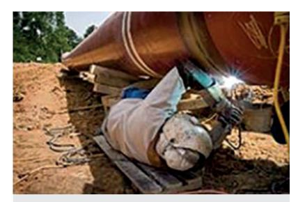
It's important to remember to never touch the electrode or metal parts of the electrode holder with skin or welding clothing and insulate yourself from the work and ground.
