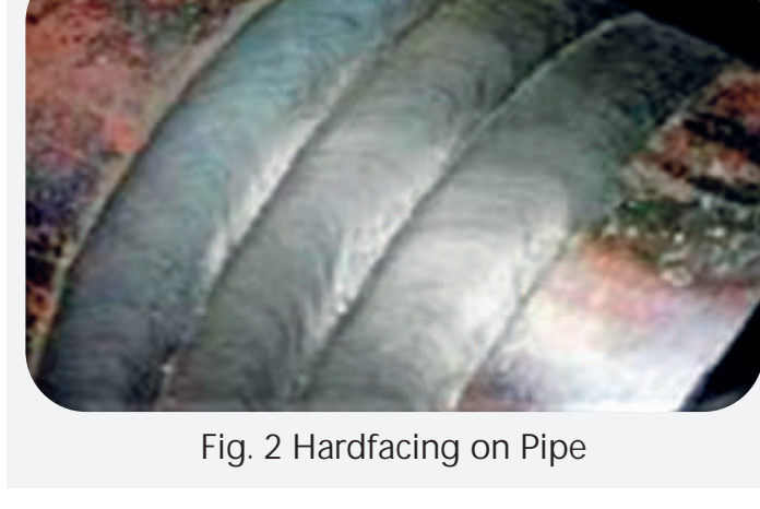
Fig. 2 Hardfacing on Pipe
