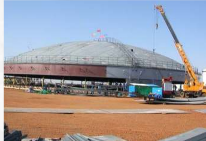
Jack-up method for Tank construction.
