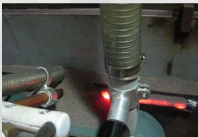
Welding in progress.
